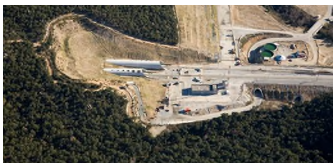
Safety facilities at Pertus tunnel South portal Spanish side (Figueras-Perpignan HS line)
