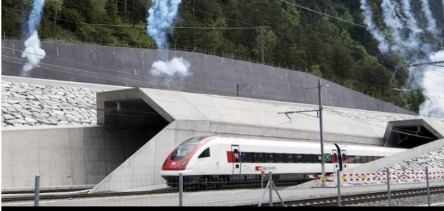
Saint Gotardo tunnel
