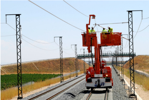
Maintenance Staff working on catenary system
