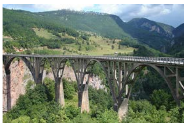
Large viaducts, made of concrete (typical length > 200m)
