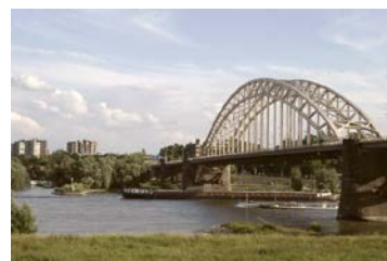
Iron bridges, mainly for crossing waterways
