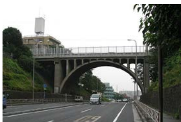
Smaller bridges, made of concrete, e.g. crossing of roads
