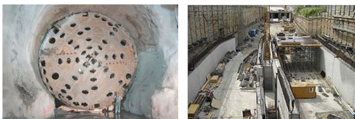
1) Tunnel in mining construction 2) Tunnel in open-pit construction
